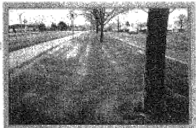
Grassy swales provide bio-filtration to help prevent pollutants in street runoff from getting into the groundwater.
