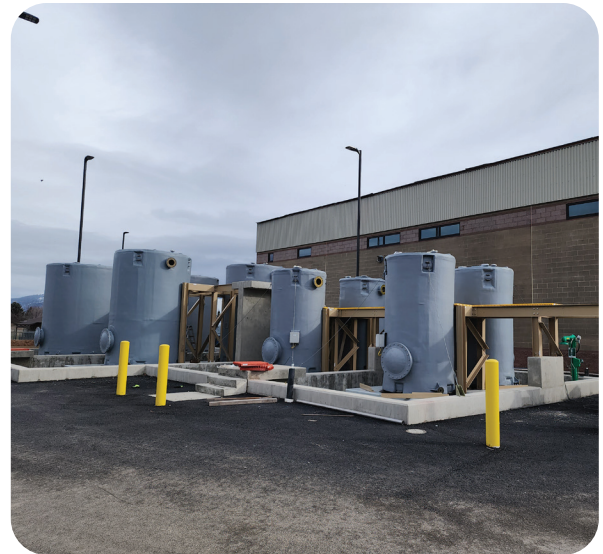
Outdoor Chemical Storage FRP tanks and Catwalk Installation (03/01/2024)
