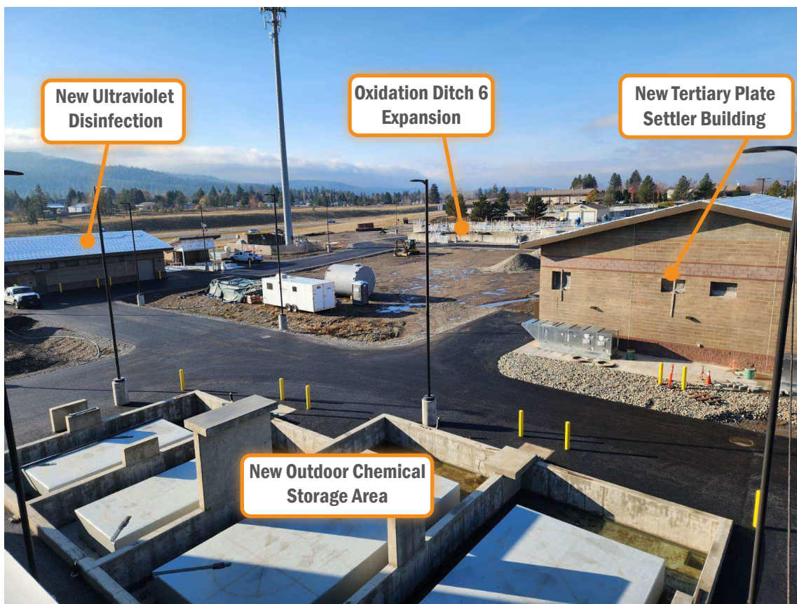
View from the Roof of the Membrane Filtration Building (looking southwest)
