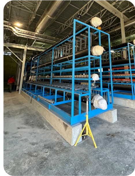
Membrane Filtration Skid Installation in the Membrane Filtration Building (10/20/2023)
