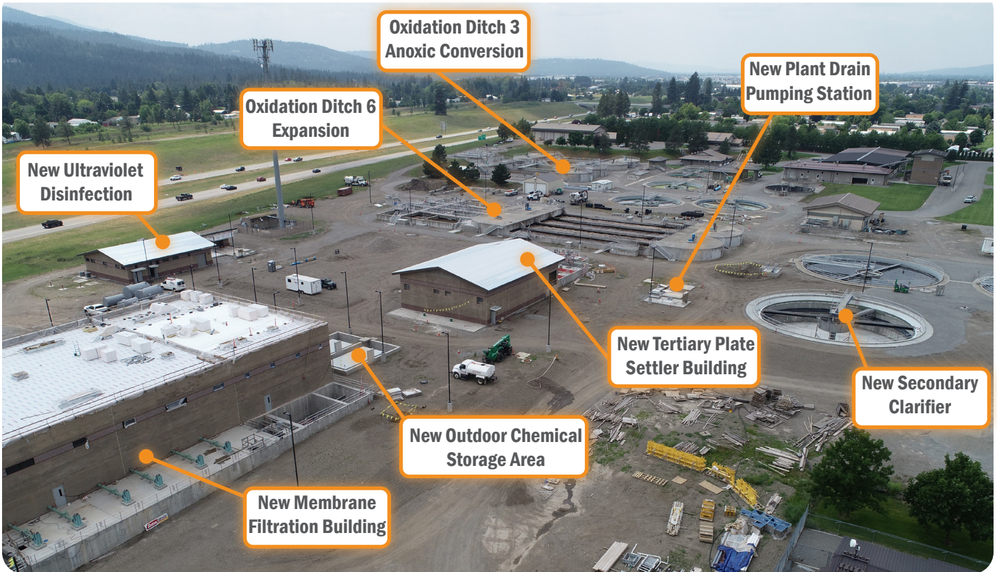
WRF Tertiary Treatment Improvements expansion area (looking south-west to I-90)
