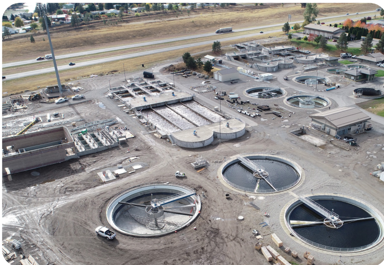
New Secondary Clarifier, Oxidation Ditch 6 Expansion, and Tertiary Plate Settler Building (10/27/22)
