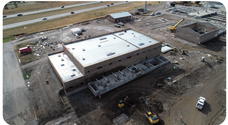
Membrane Filtration, Tertiary Plate Settler, and Ultraviolet Disinfection Buildings (10/27/22)
