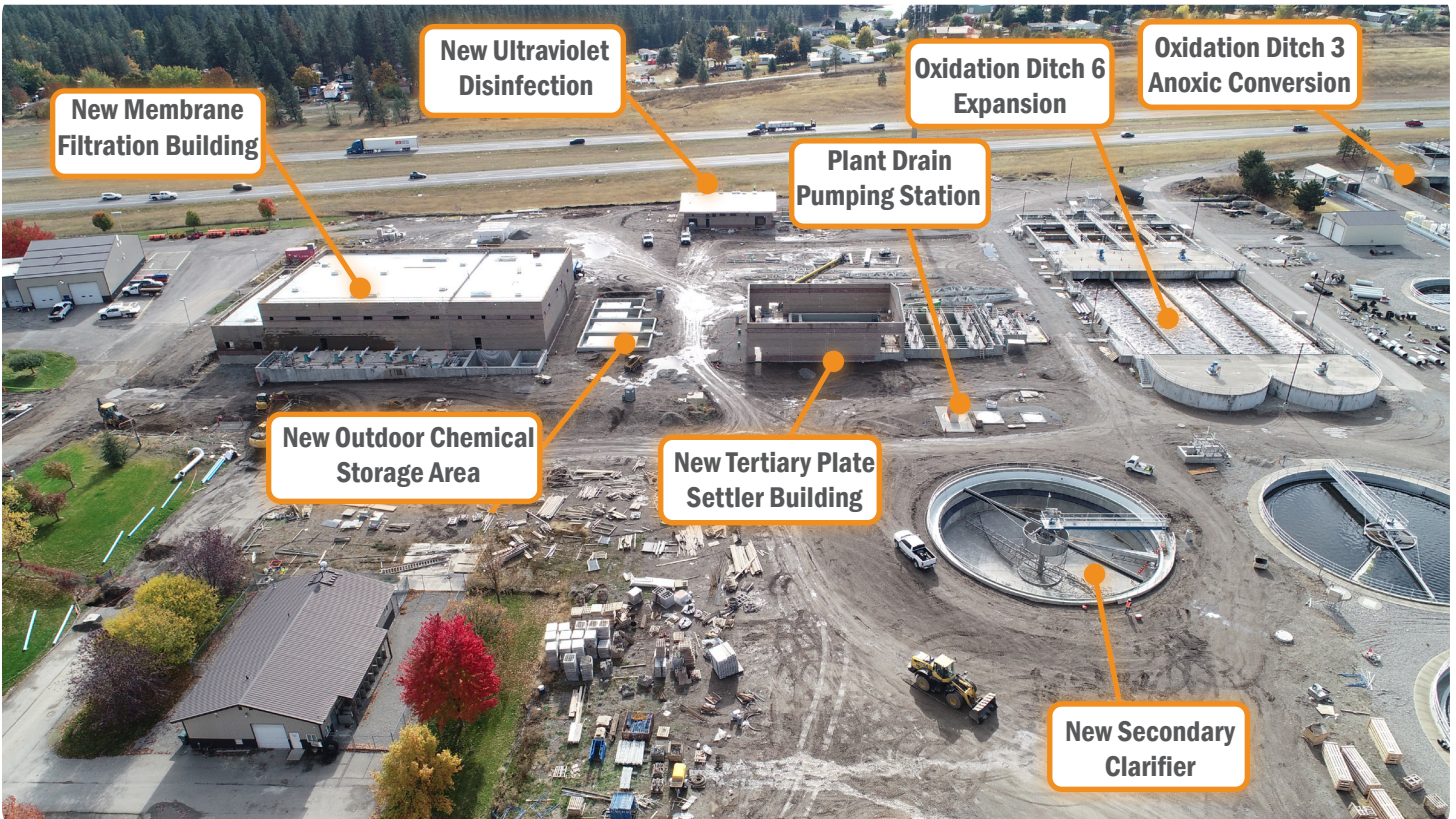
WRF Tertiary Treatment Improvements expansion area (looking south-west to I-90)
