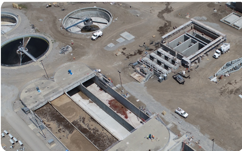
New Secondary Clarifier, Oxidation Ditch 6 Expansion, and Tertiary Plate Settler Building (7/9/22)
