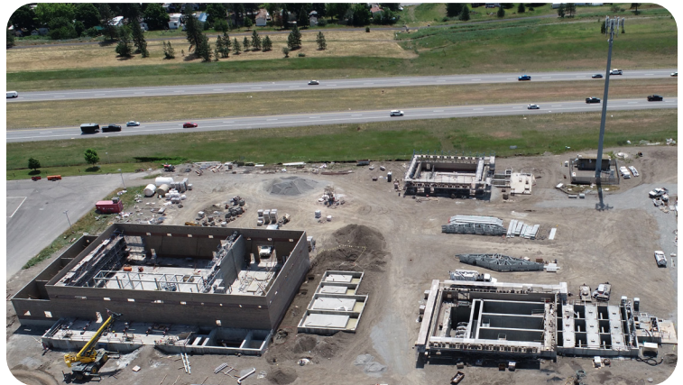
Membrane Filtration, Tertiary Plate Settler, and Ultraviolet Disinfection Buildings (7/9/22)
