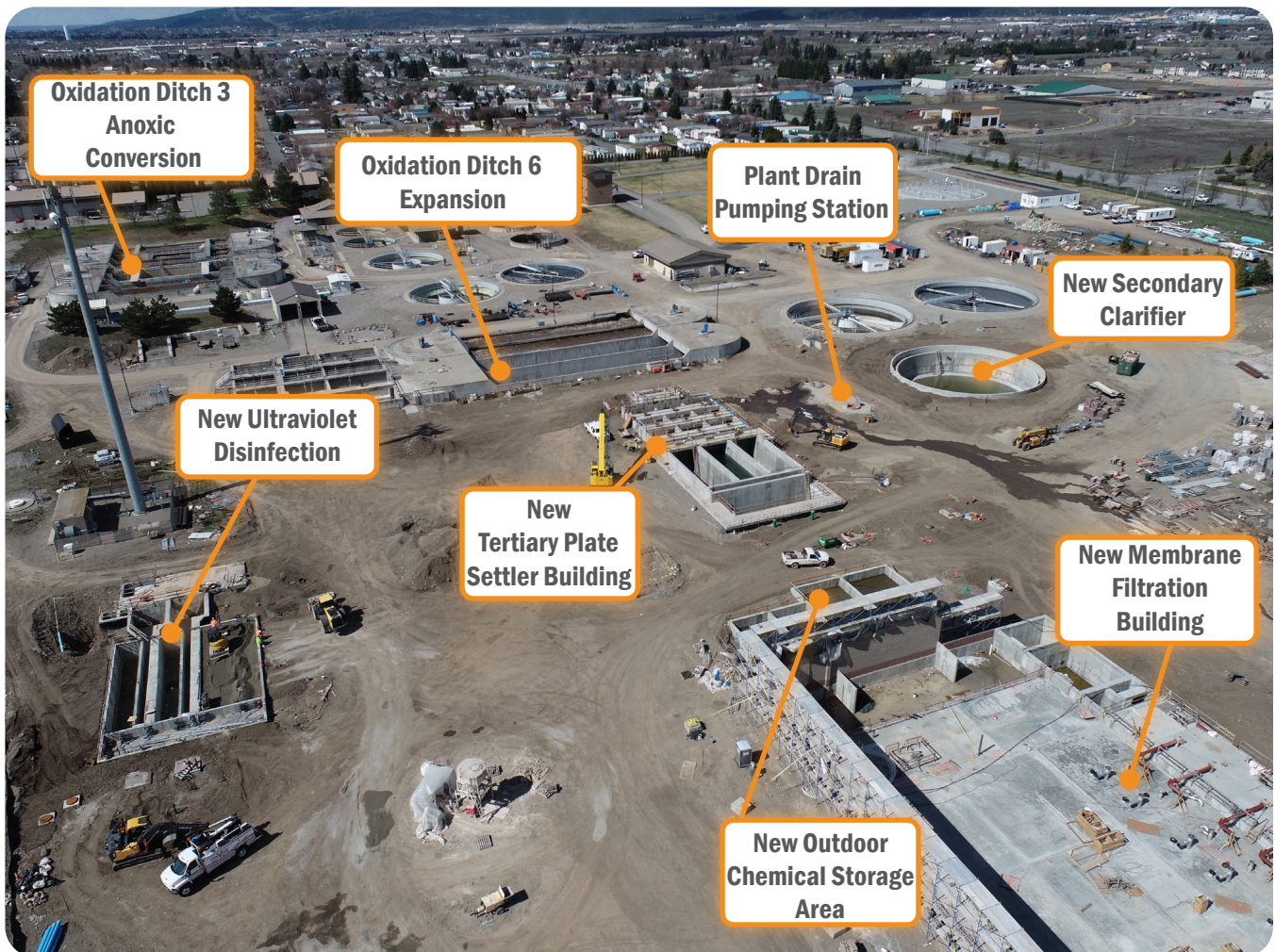
WRF Tertiary Treatment Improvements expansion area (looking north-west to Seltice Way)
