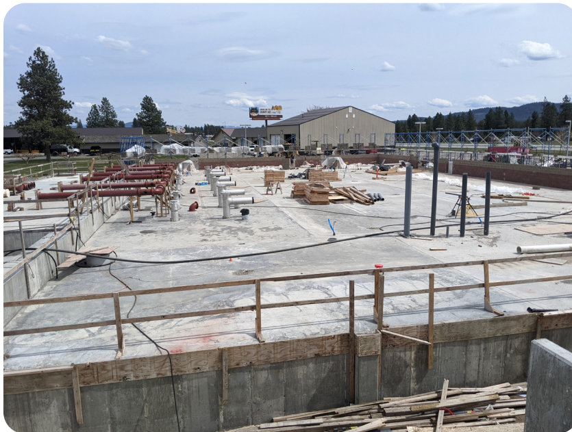
Membrane Filtration Building (4/25/22)
