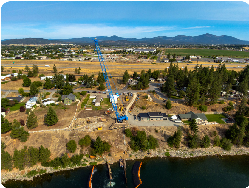
Spokane River and WRF Outfall Pipeline Corridor (8/26/21)
