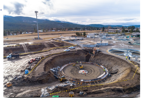
Secondary Clarifier No. 8 underslab piping and concrete foundation formwork (1/5/21)
