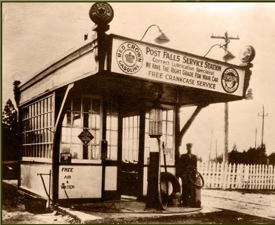
ABOVE: This Red Crown service station was one of the earliest gas stations in Post Falls
