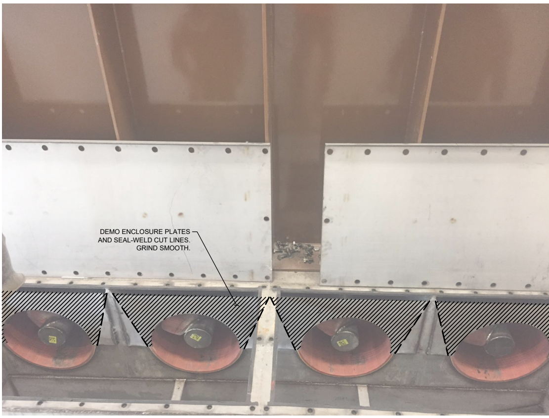
5 DEMOLITION PHOTO DETAIL SCALE: NOT TO SCALE
