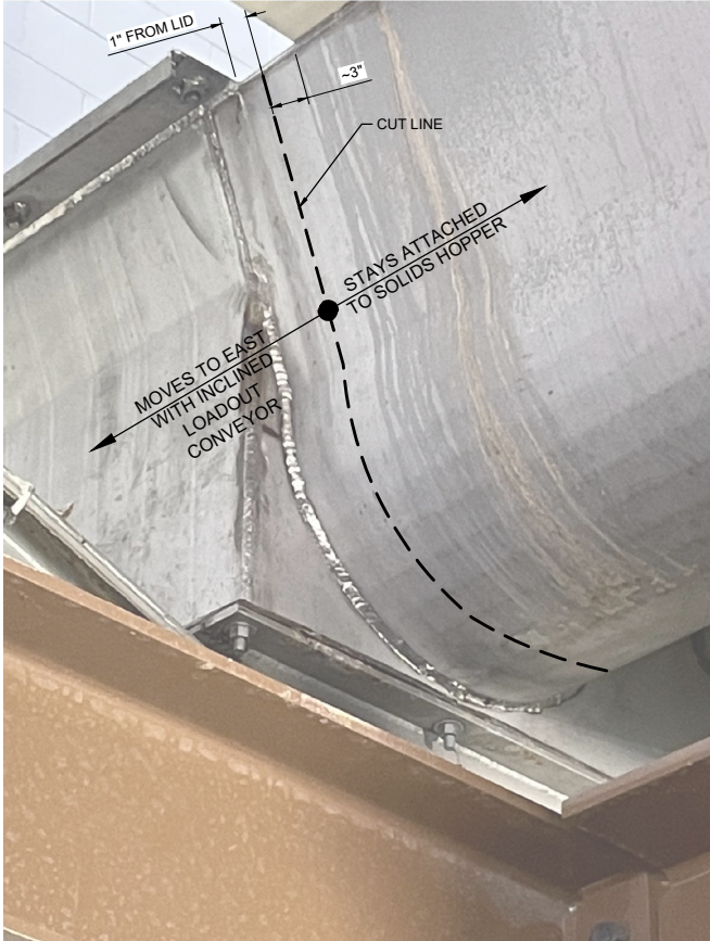
2 DEMOLITION PHOTO DETAIL SCALE: NOT TO SCALE
