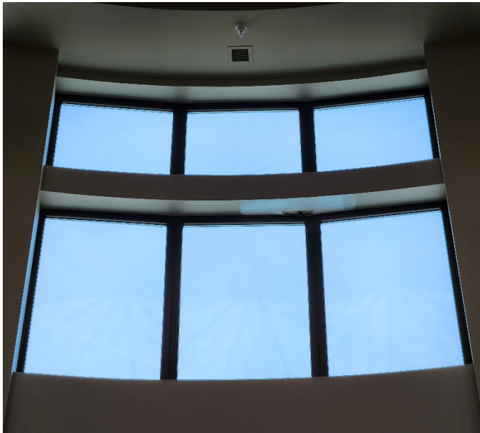
Photo #4: Close up of Rotunda drywall damage.
