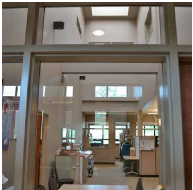
FIGURE 91. LIGHT WELLS DAYLIGHT TO BUILDING INTERIOR
