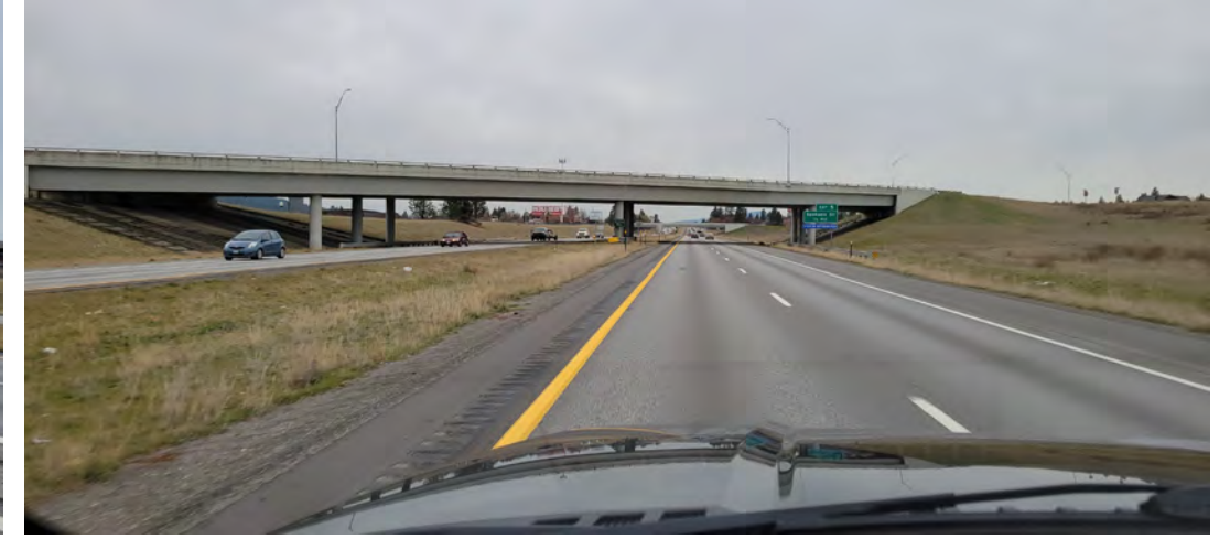
1-90 Westbound - Seltice Way Overpass
