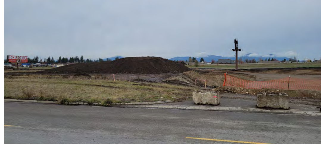
Access Drive at 4th Avenue Looking North
