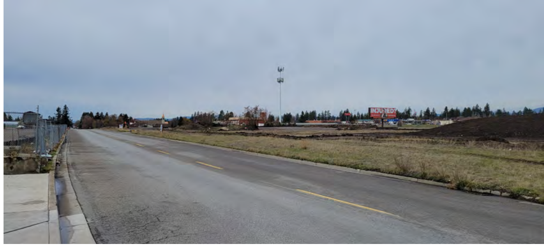
Access Point at 4th Avenue Looking West
