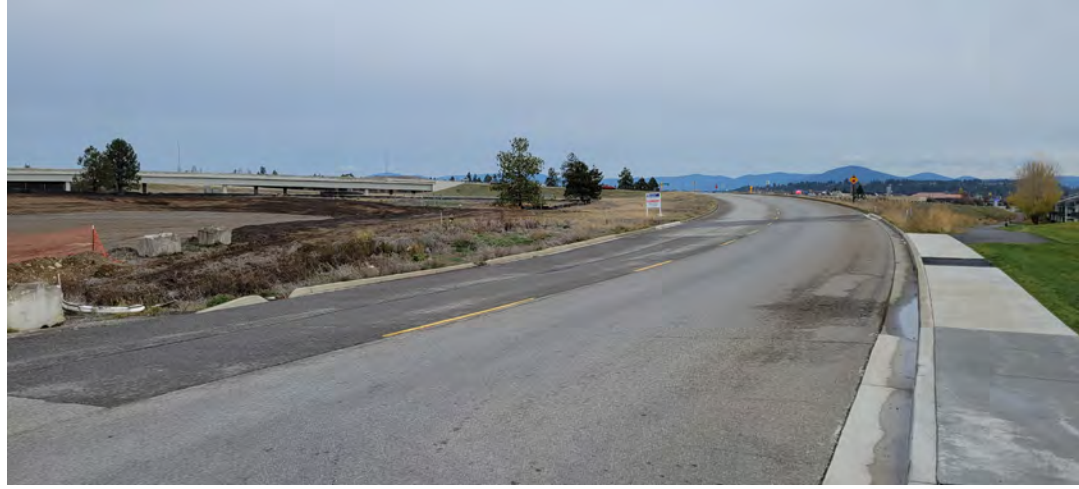
Access Point at 4th Looking East
