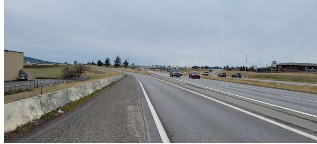
Eastbound 1-90 On-ramp at Seltice Way Looking West
