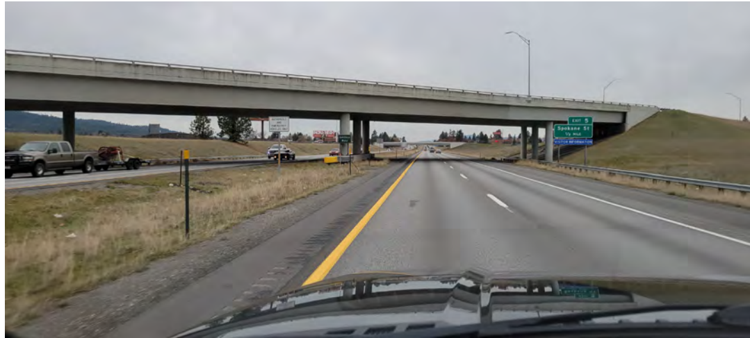
1-90 Westbound - Seltice Way Overpass
