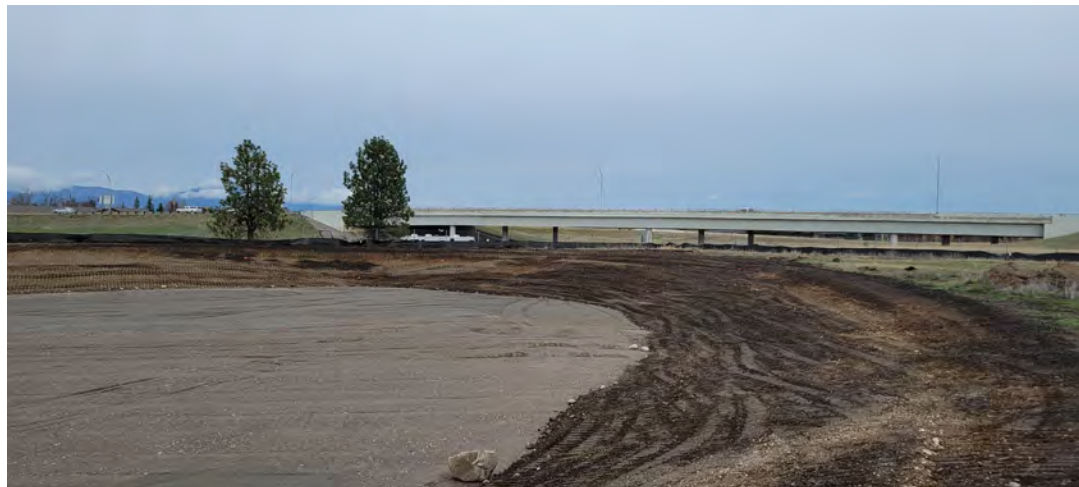
Current Site Grading
