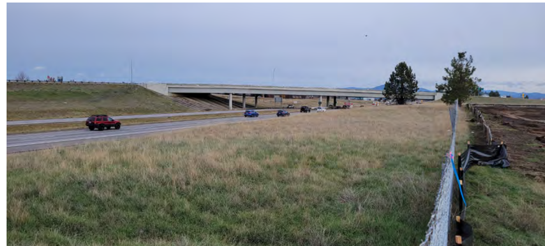
North Edge at 1-90 Looking East
