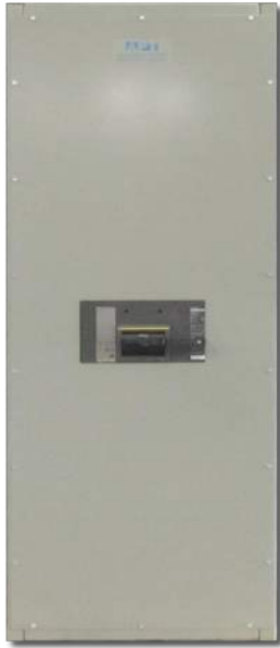
Figure 7: 1 MW, 480V, 1600A Generator Disconnect & Output Protection Molded Case Circuit Breaker with Front Removable Sheets
