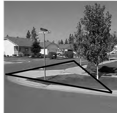
Figure 7 – Vision clearance A vision clearance triangle is 40' from the intersection's road or curb edge.
