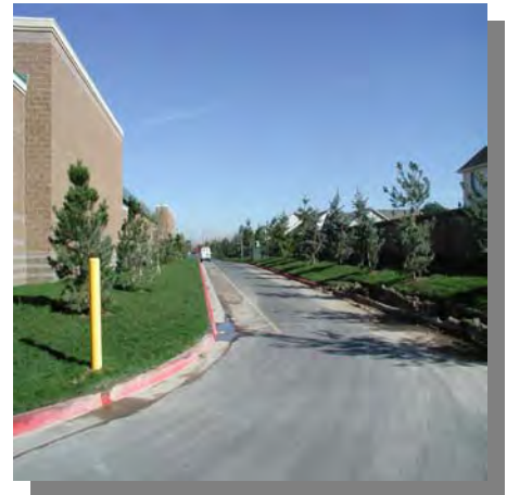
Secondary Access Road
