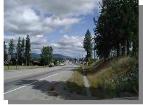
Highway 41 looking north to Mullan Avenue
