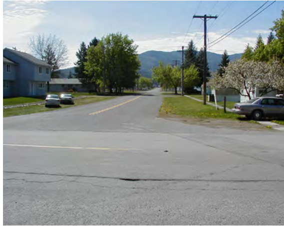
Right-of-Ways on north/south streets between 5th and 3rd offer opportunities for widening and addition of street parking
