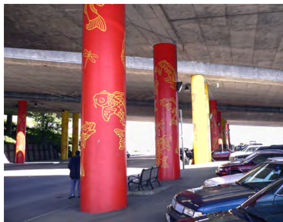
Freeway Columns Used as a Canvass for Public Art
