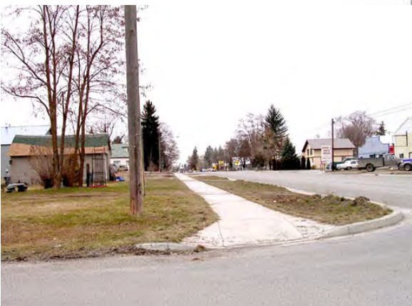
Recent sidewalk improvements along 3rd Avenue
