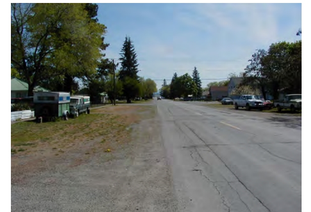
4th Ave. is over-due for structural re-construction to the city's major collector standards.
