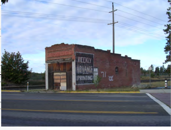
Currently vacant building with historic character
