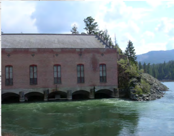
The Avista dam is an important historic resource
