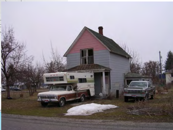
Empty house on 2nd Avenue used for storage
